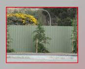
BHP COLORBOND® steel sheeting and capping with galvanised metal posts and rails. This fencing is only coloured on one side.
